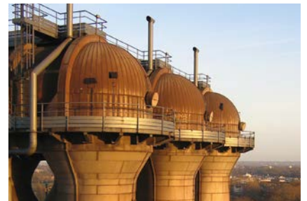
Blast furnace / stove dome
